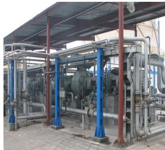
**Coke oven gas compressor for steel mill**
